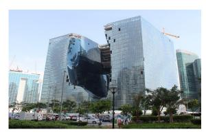
The Opus, costing AED 2.5 billion consists of two glass towers linked by a four-storey podium at ground level, and at a height of 71 meters by an asymmetric steel and glass bridge. With an organic void right at the heart of the building, The Opus has 56,000 square feet of office space, 12 restaurants and a five-star boutique hotel with only 93 guest rooms and 60 apartments.
